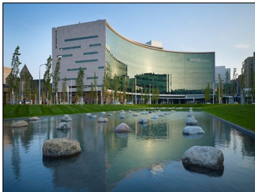
Figure 2: Cleveland Clinic, Ohio, USA
